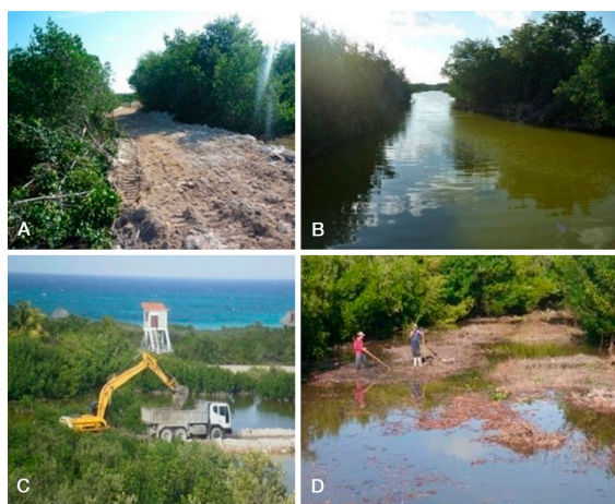
Fig. 1. – Some restoration implemented actions at Laguna Larga between 2010 and 2012. A, filling of road to dredge the channel; B, dredged channel; C, dredging of channel at the central section; and D, cutting of red mangrove roots.
