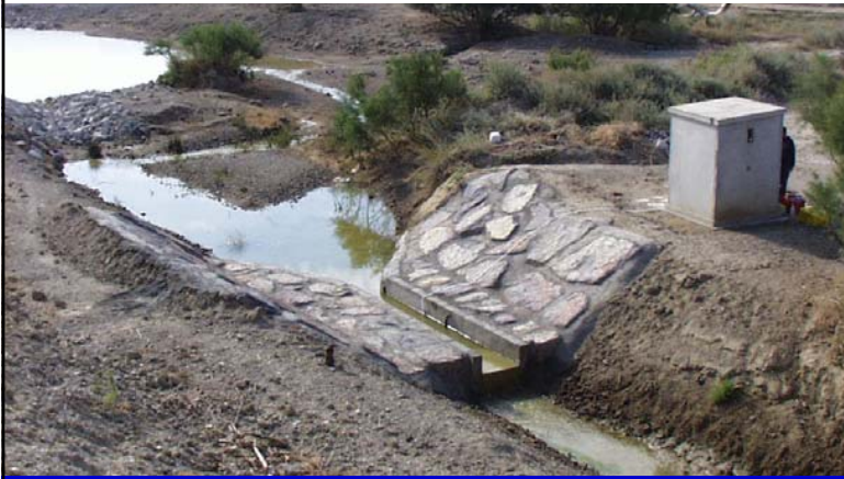
Flow and quality station in Lerma (Bardenas)
