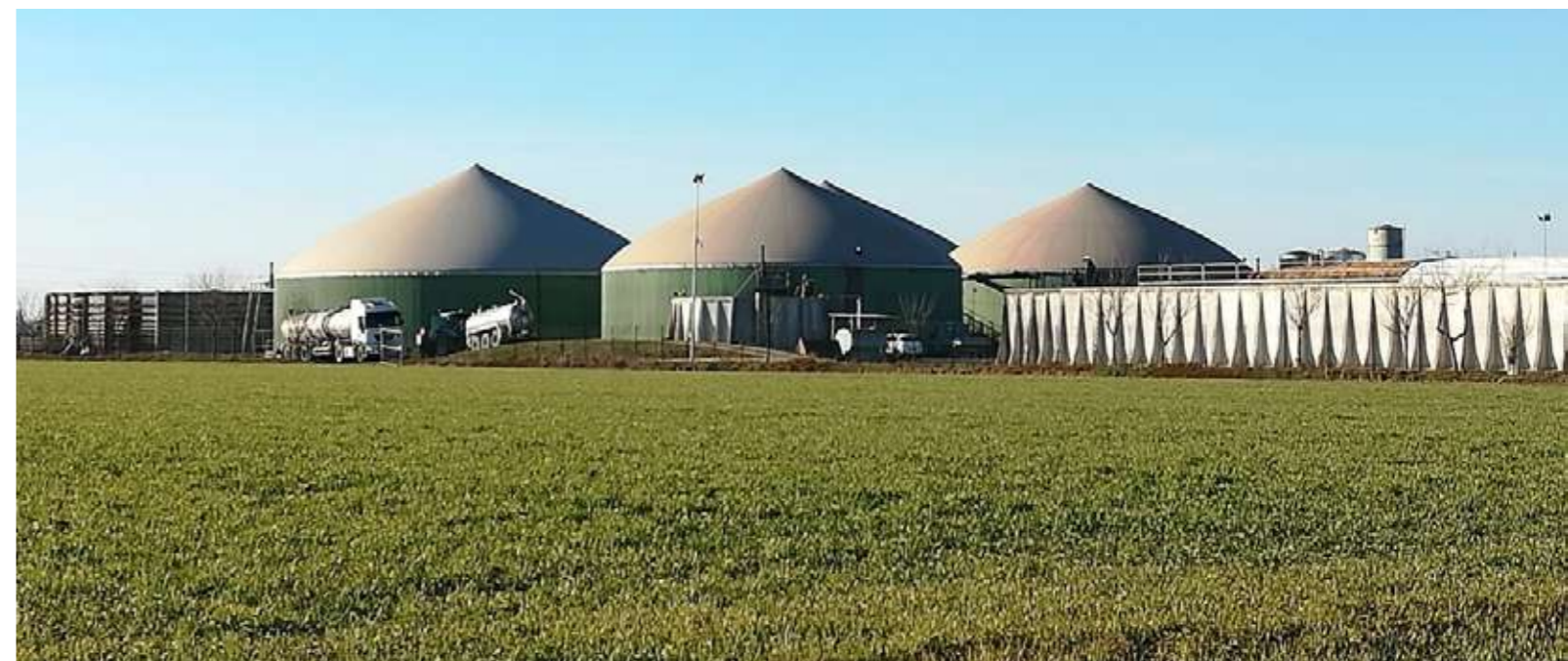
Image 3.10. Anaerobic digestion plant in Lombardy.
