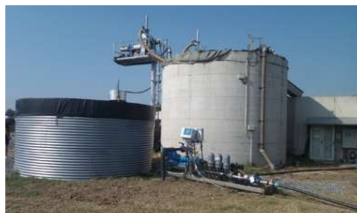
Image 3.7. Direct injection of digestate liquid fraction from the farm storage tank in the irrigation system.
